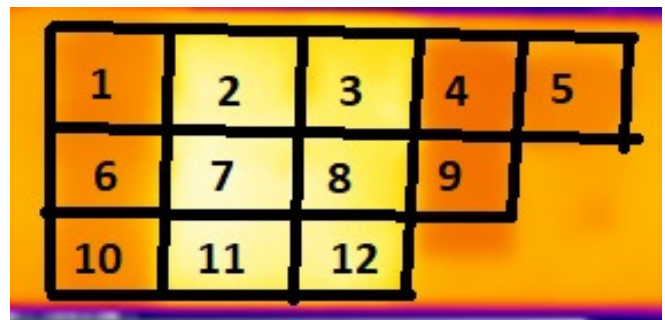
Thermal image facing sun - from back
